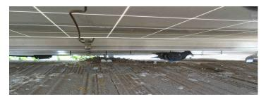
The best way to address this problem is to install bird deterrents, ideally when solar panels are first installed, or at the very least before pest birds arrive.
